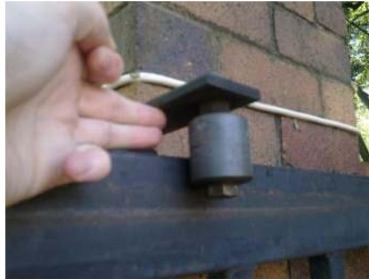
Make sure the anti-lifting bracket is installed as close to the gate as possible. In the above example, the gap above the gate is too big, the gate can still be lifted. The gap must be less than 1cm
