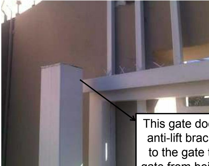
This gate does not have an anti-lift bracket welded on to the gate to prevent the gate from being lifted on the side of the gate motor.
