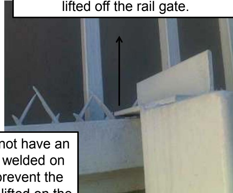
Gate with an anti-lift bracket fitted to prevent the gate from being lifted off the rail gate.
